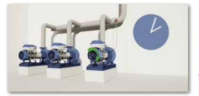
Alternate work to maximize each pump lifespan
